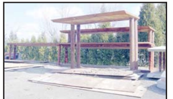
TRENCH BOXES AND ROAD PLATE
